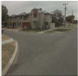
A) Unlined basic intersection
