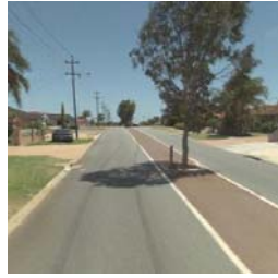
Painted median with occasional island: extra wide lane accommodates car and bike side by side
