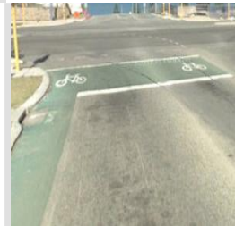
H) Head start facilities
